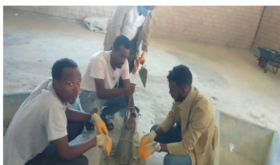
a) Measuring result of slump test
