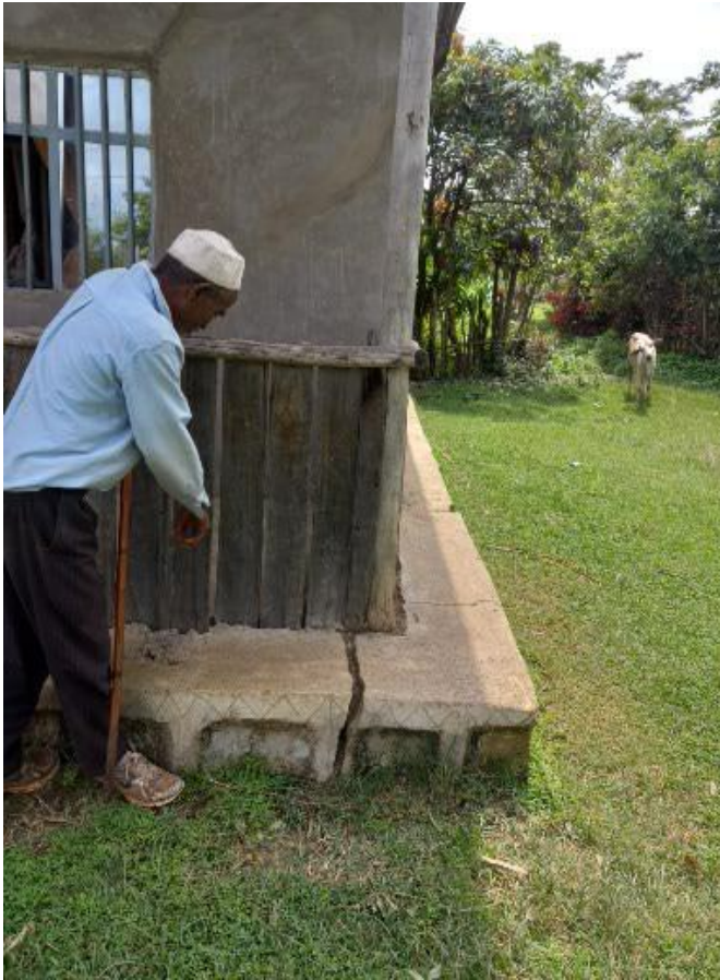
Fig. 4.8 cracks in the houses of residents
