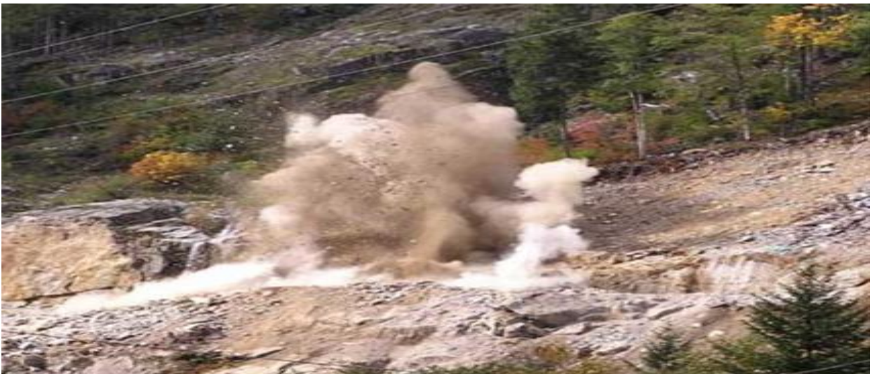
Fig. 4.10 blasting in Gibril hairu Construction Materials manufacturer site
