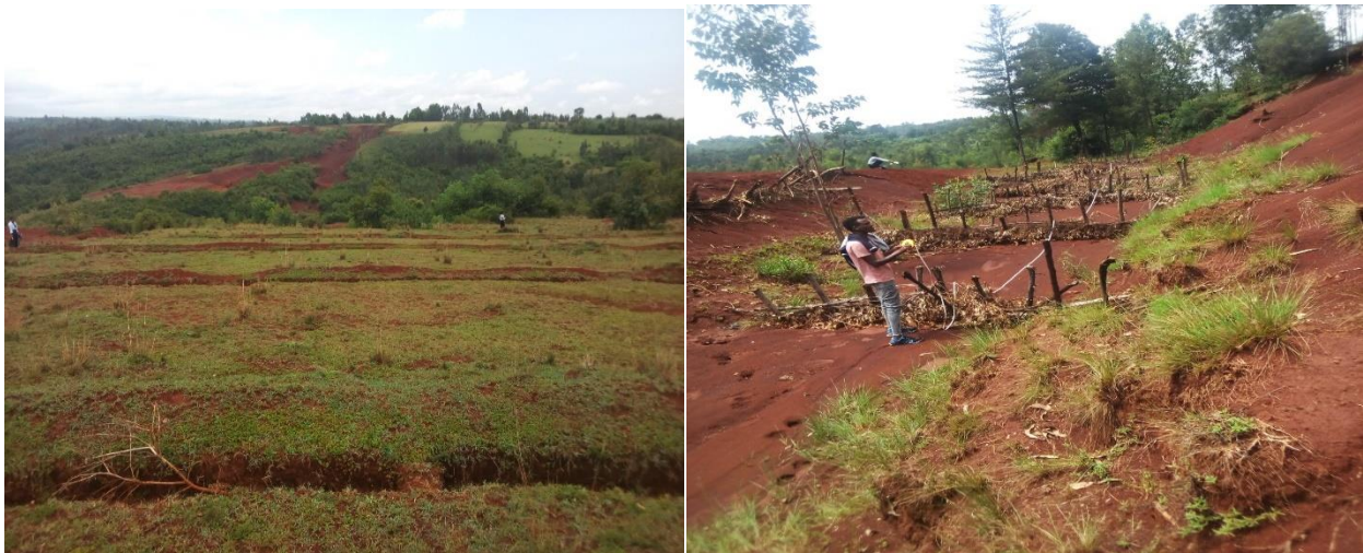
Figure 4: Structure of level soil bund and brush wood check dam
