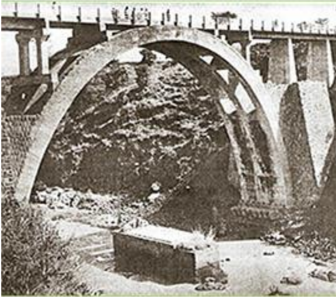
Figure 4.4.9. Building of Roads
